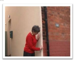
and rear walls were insulated externally, giving a smart rendered appearance. "Breathable" products and brick effect finishes are also available. The work was quite disruptive and noisy, with scaffolding outside and radiators and skirtings needing to be
